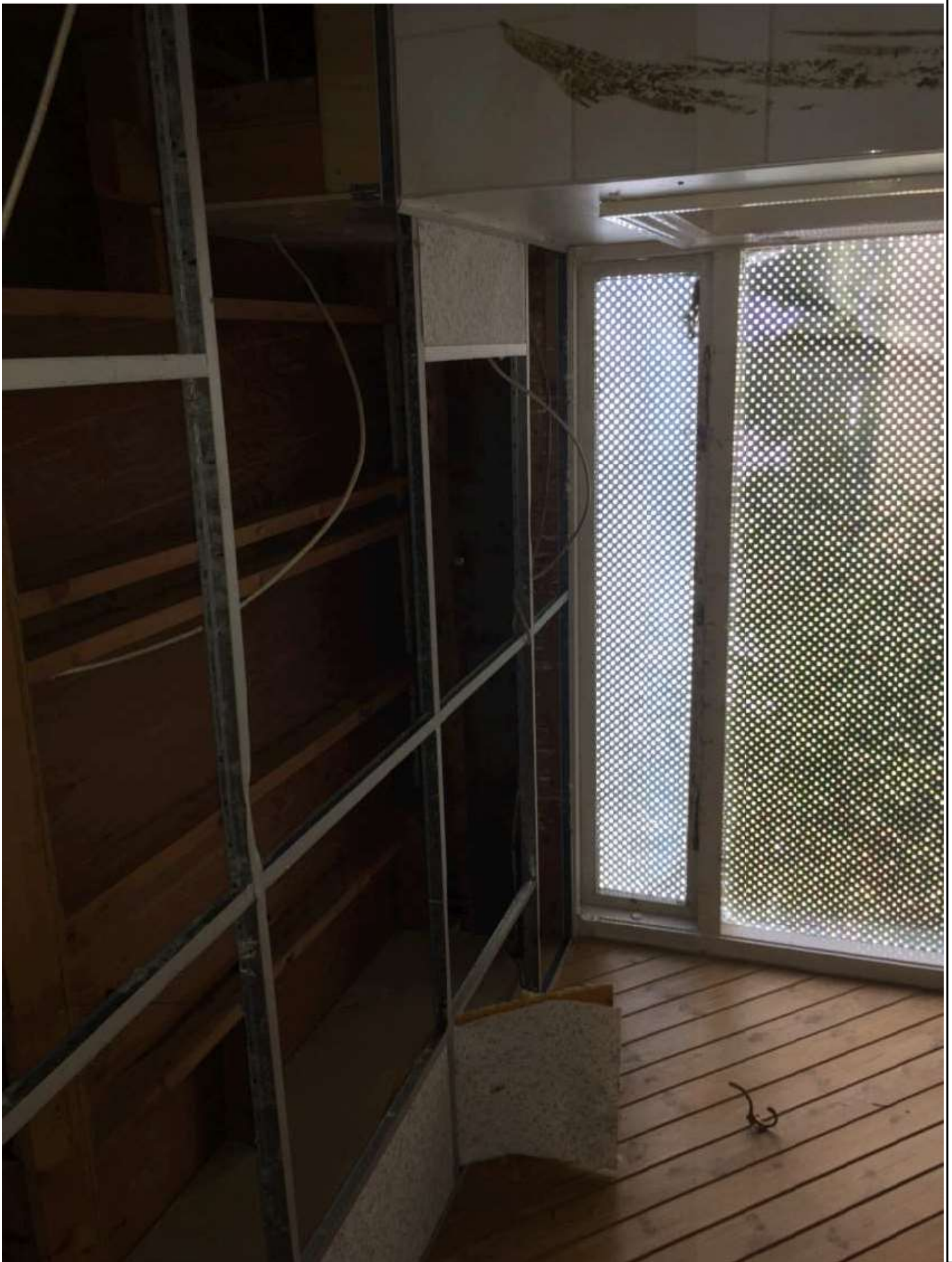
Image showing the internal condition of the building - image 4
