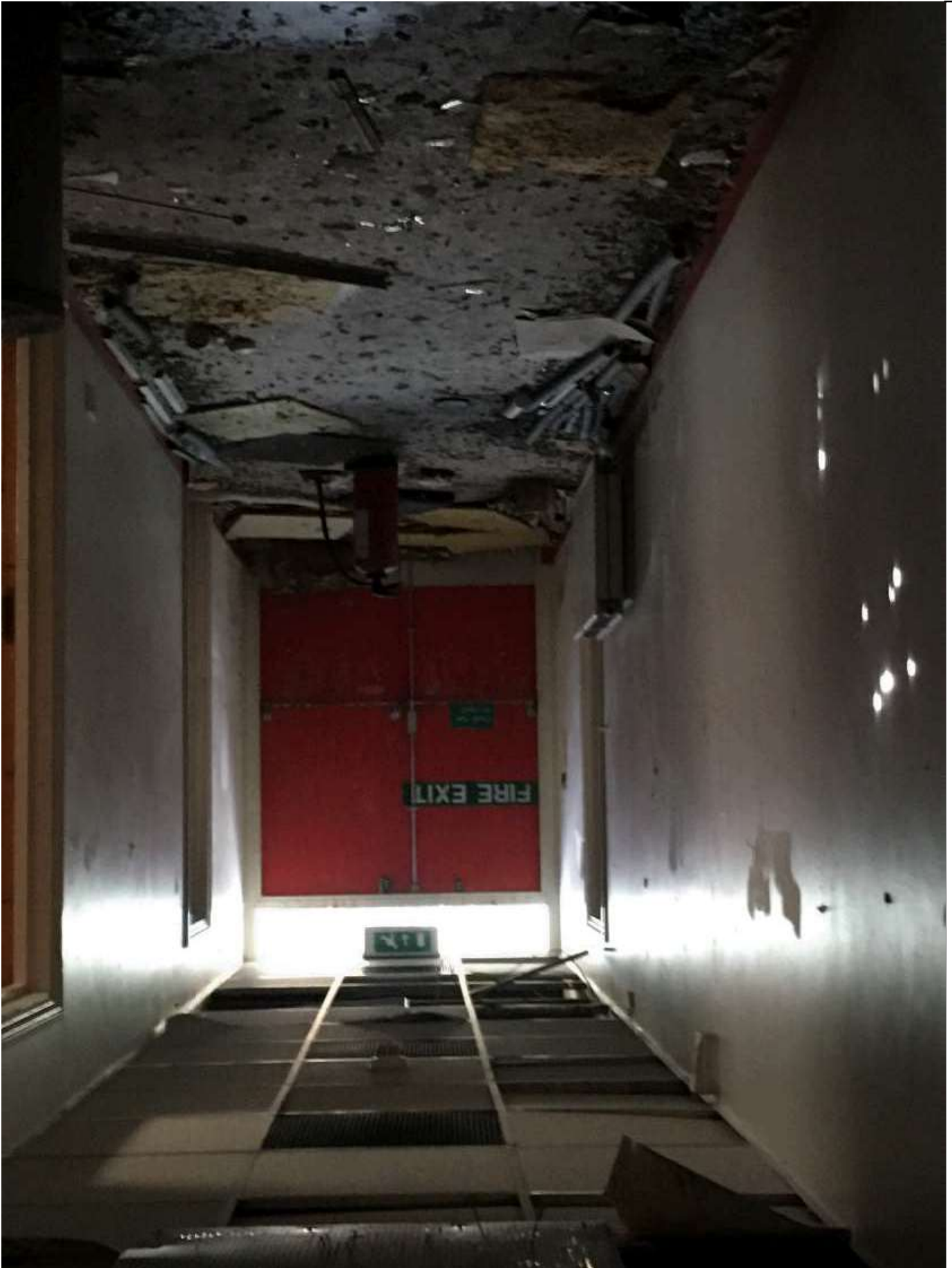
Image showing the internal condition of the building - image 1
