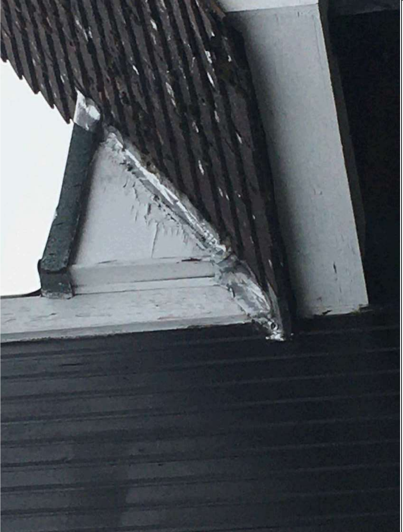
Image showing the condition of the building and its tiled roof
