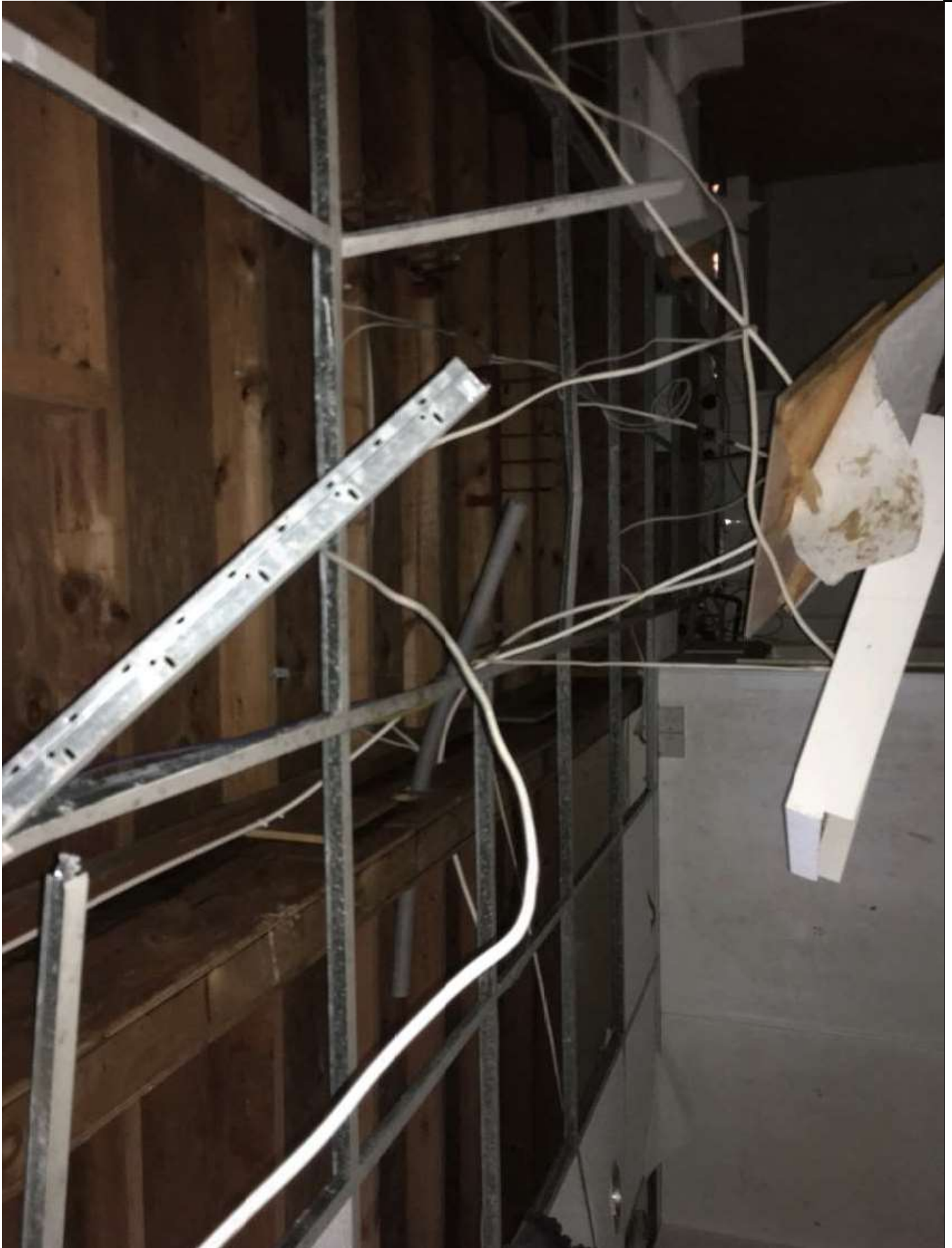
Image showing the internal condition of the building - image 2
