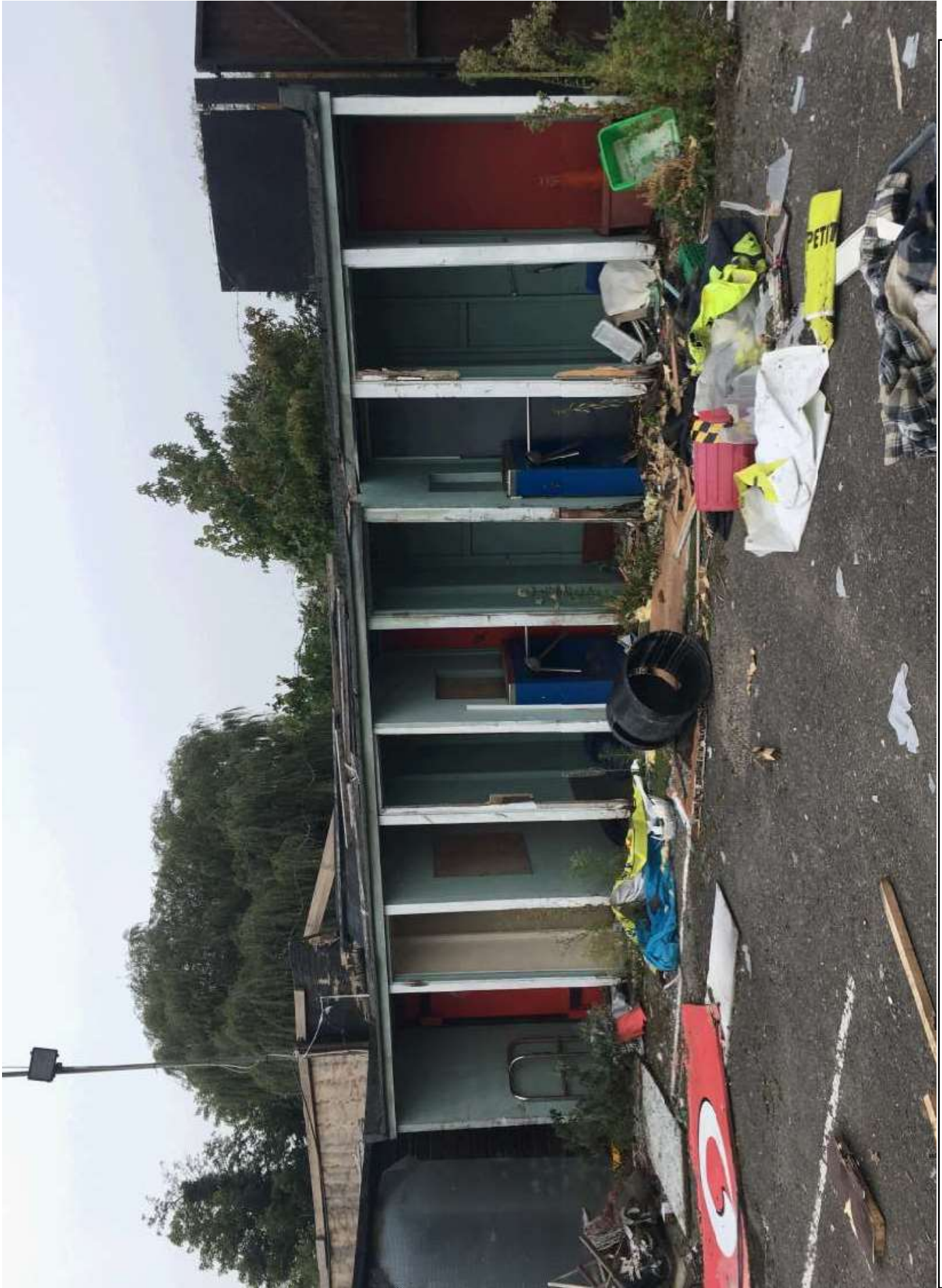
View of the turnstiles to be demolished
