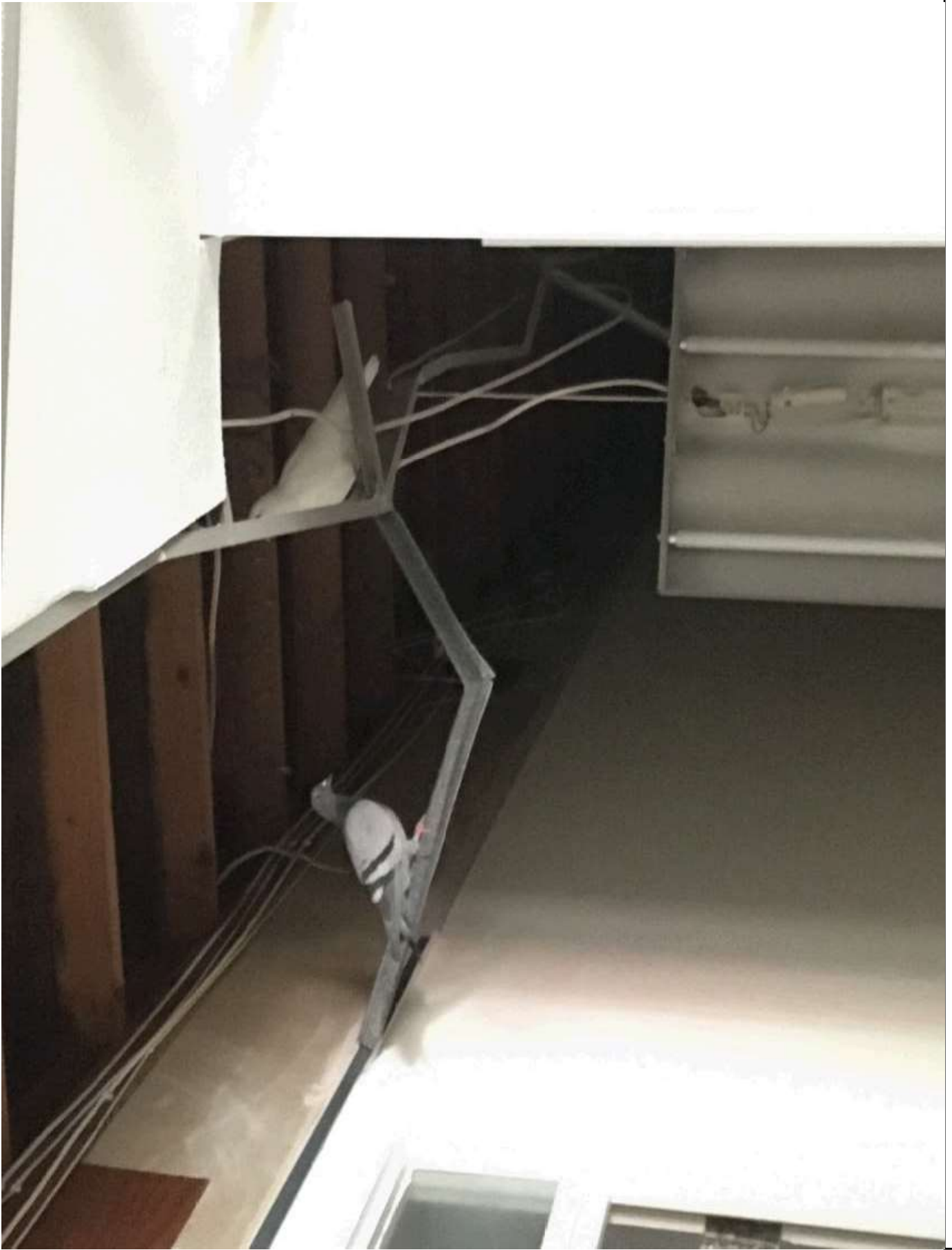
Image showing the internal condition of the building - image 5
